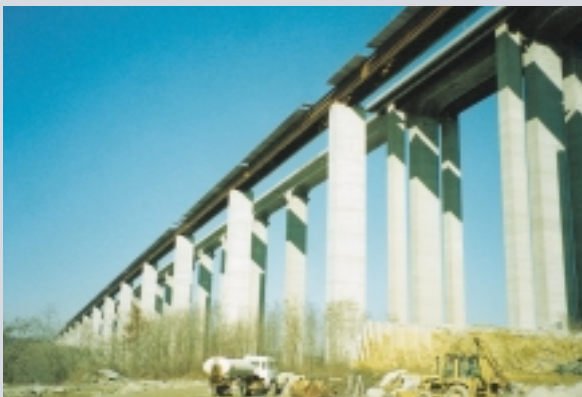
Stura di Demonte, Italy built: 1999 Composite steel bridge length of bridge: 2750 m type of joint: DS1200 24.50 lin. metres
